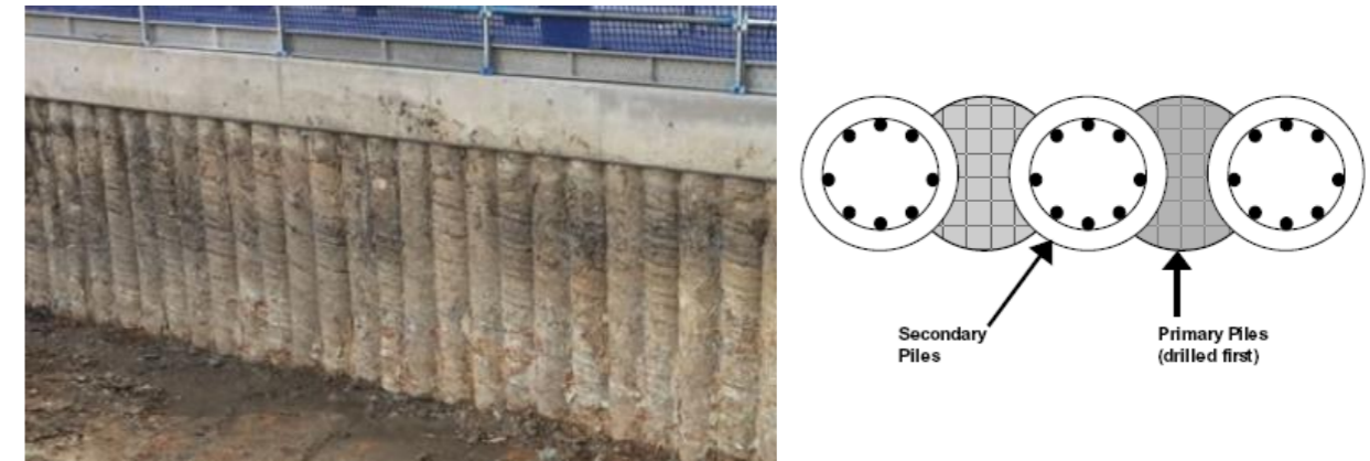
Figure 17. Secant piles structure solution
